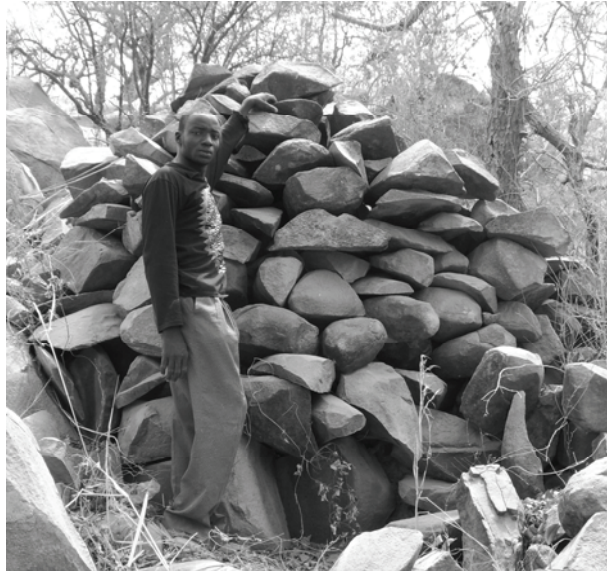
Figure 3: Cicipu speaker Mohammed Mallam standing by a well-preserved section of the fortified wall surrounding Korisino (Karishen) hill, near Sakaba
